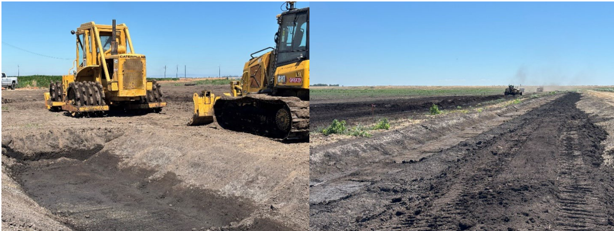
Figure 10.1. Heavy equipment staging and site prep for wetland construction on Staten Island. Photos taken by J. Dixon on July 7, 2026.
