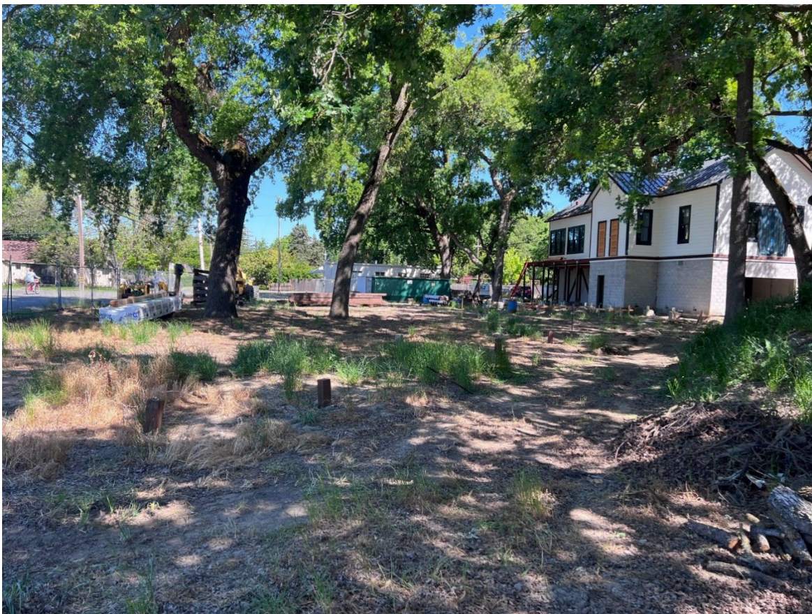
Figure 9.1. Acquired property with schoolhouse under construction.
