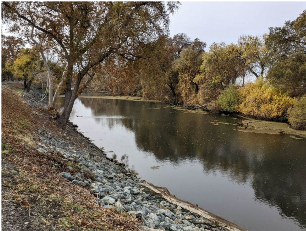
Figure 7.2. Riprap on the left bank of Elk Slough.
