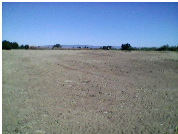
Figure 2. Ulatis Creek habitat restoration site after ground preparation activities.
