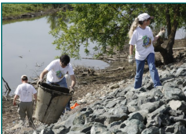
“Bucket Brigade” used on steep levee banks
